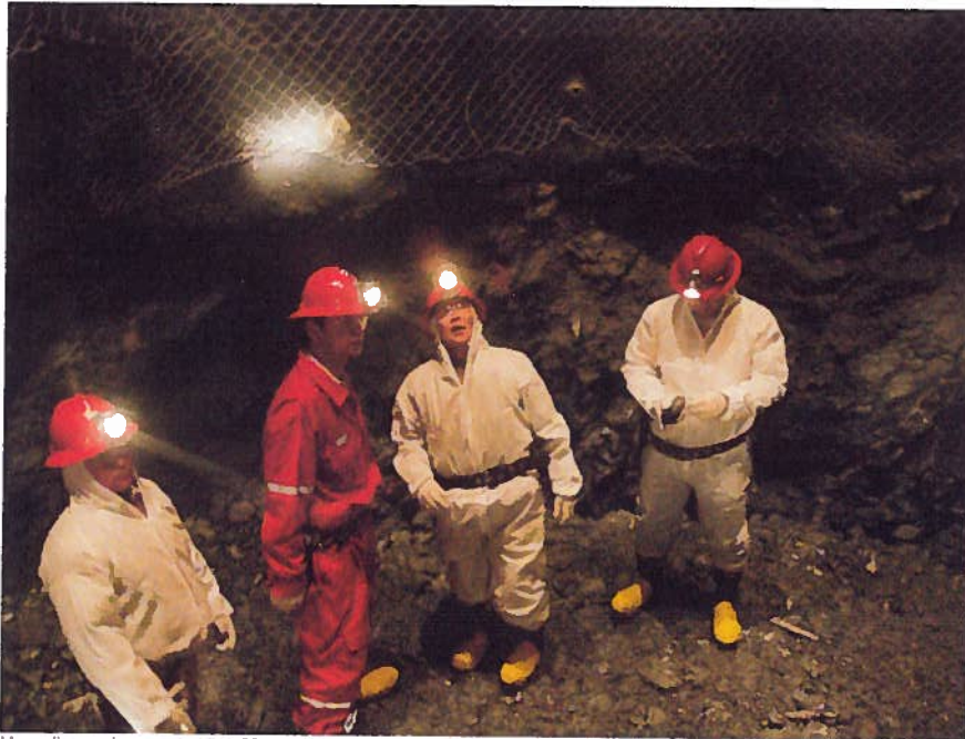
Mongolian workers are seen at 551 meters below the surface of the earth while sinking an exploration shaft at the Oyu Tolgoi copper-gold project
